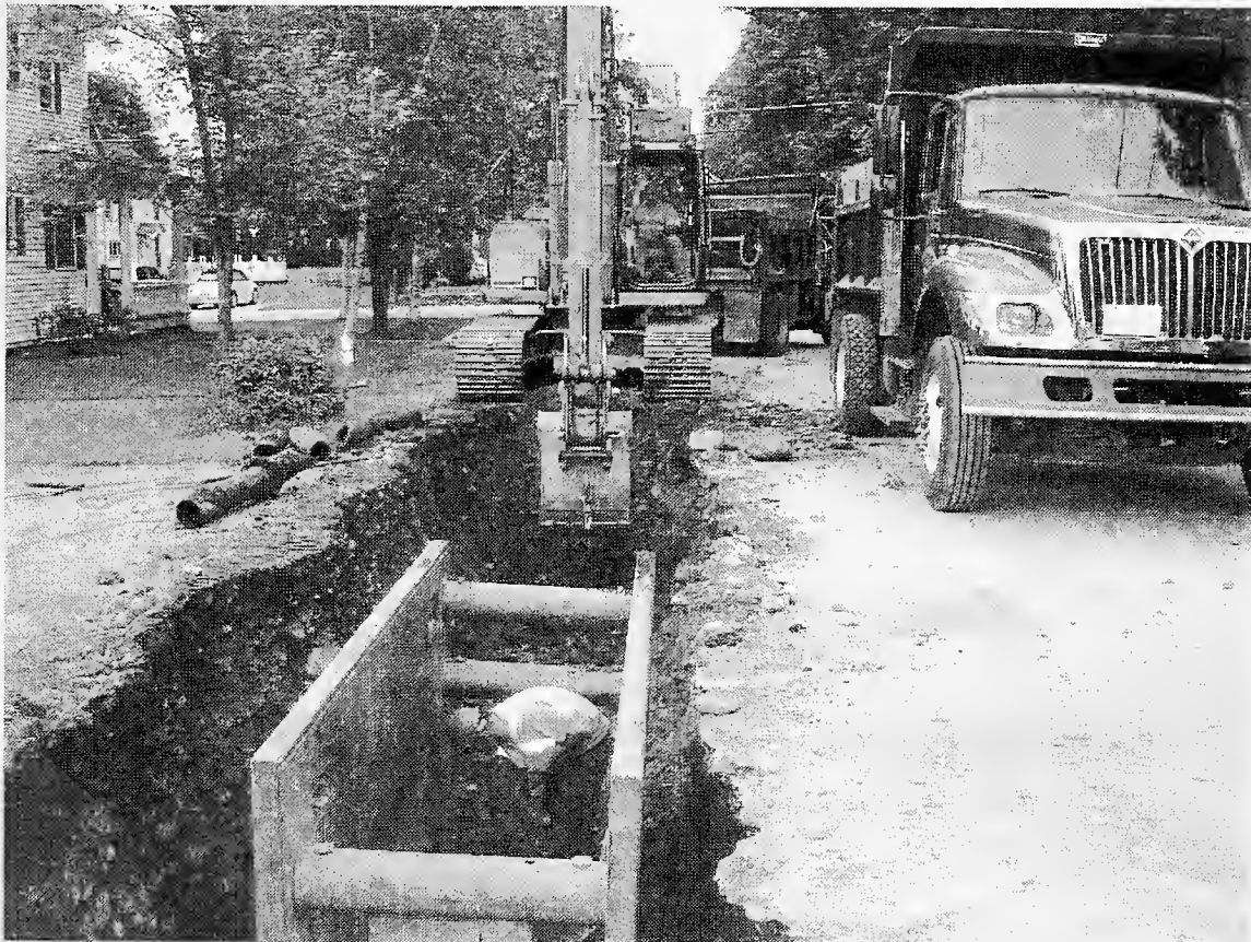
Installation of new 8-inch ductile iron water main on McFarland Street.
